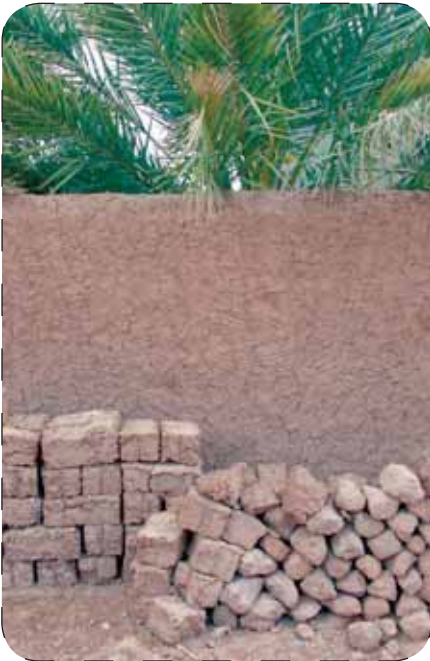
Molded blocks and adobe made of mud
