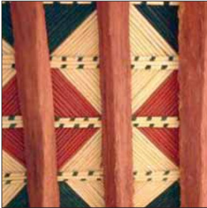
Type B floor (beams and oleander rods)
