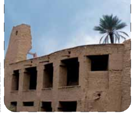
The wall of the Ajdir plaza, before and after restoration
