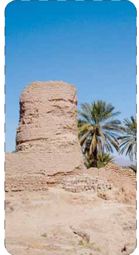
Figuij, earthen watchtower
