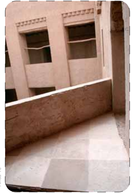
Africa 70 Saving the heritage: house being restored
