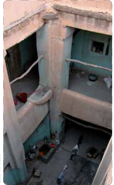
Courtyard and gallery of Figuig homes
