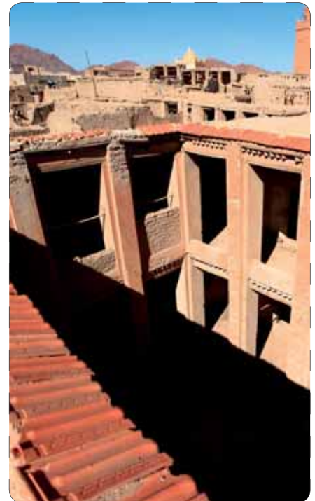
Terracotta tiles protect the parapet
