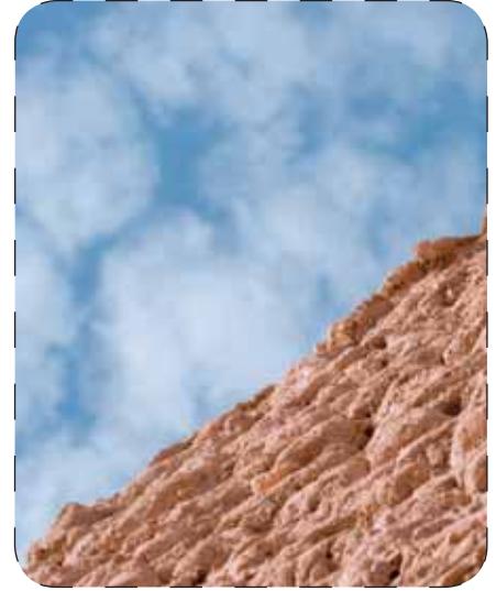
Old structures deteriorating
